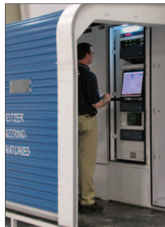
Prewired and factory tested termination cabinet for quick commissioning.
